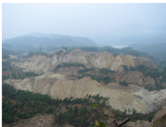
Fig. 3 Gigantic land slide at Aratozawa dam. After Chigira (2008).
