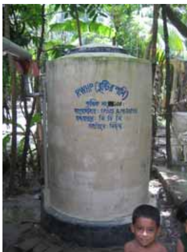
Picture 1 Rainwater harvesting tank at household level, Morrelganj
