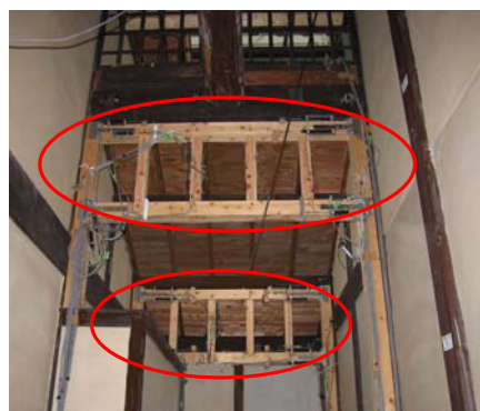
Photo 6 Seismic reinforcement using laddery frames
