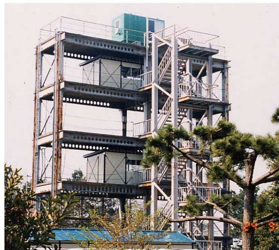
Photo 2 Full-scale five-story steel building
