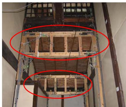
Photo 6 Seismic reinforcement using laddery frames
