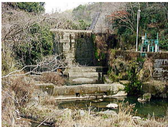
Photo 1 A photograph of check dam in the Kurama River
