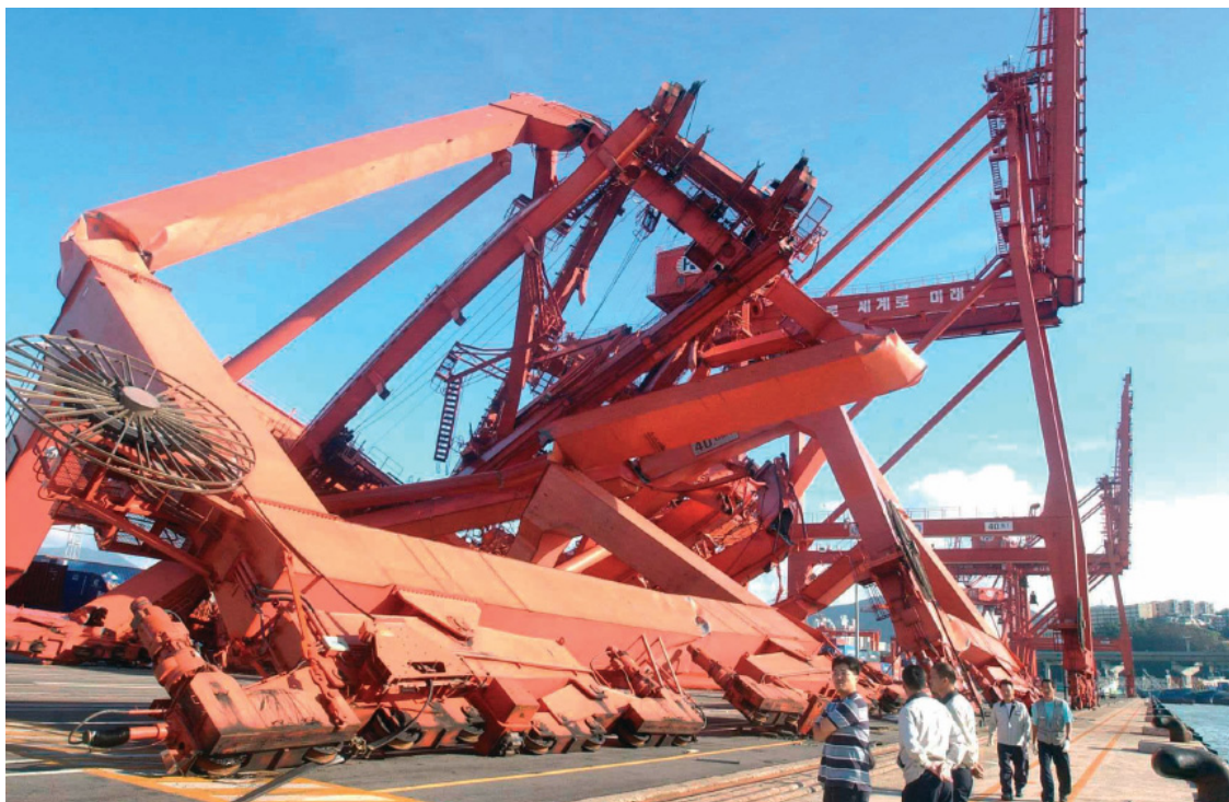
Fig. 3 Container cranes in Pusan port destroyed by strong wind during Typhoon Maemi
