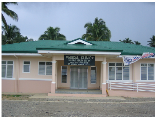
Photo 6 Barangay medical clinic at relocation site in Magbagacay-brgy.
