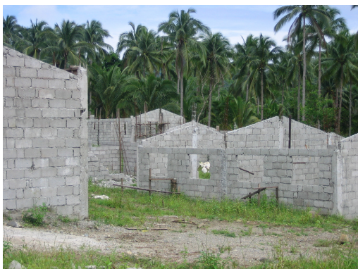
Photo 8 Housings still under construction in Catmon relocation site. .
