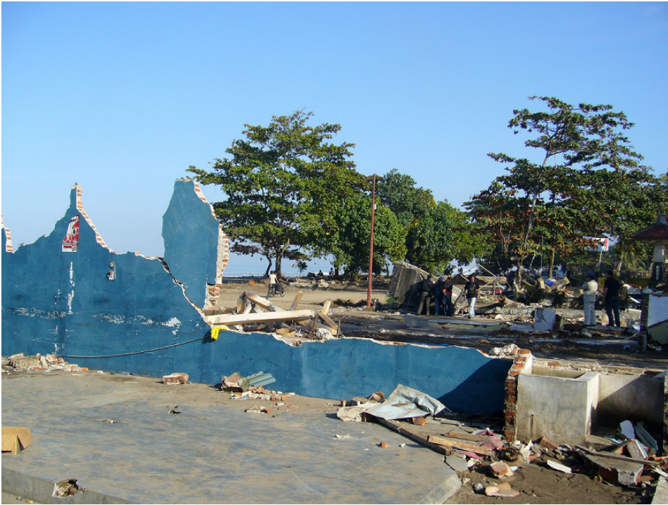
Fig. 4a Tsunami damage to unreinforced masonry buildings and debris in Pangandaran.
