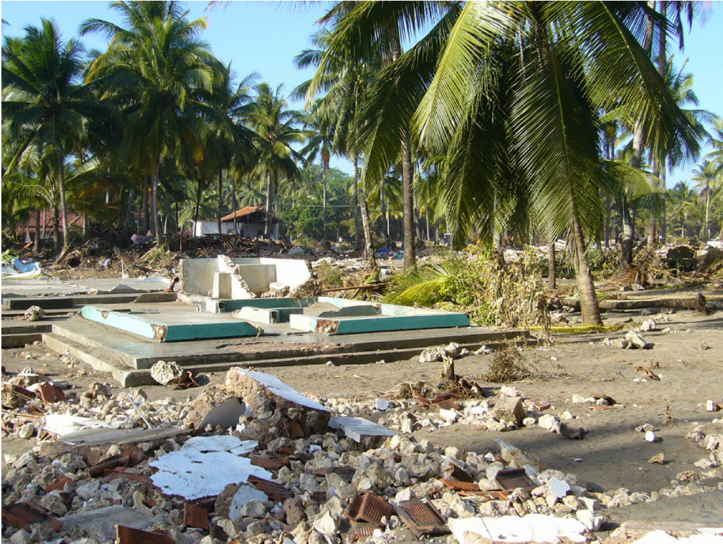
Fig. 5 Severe damage in Marsawah village where no walls were left standing for buildings within about 150 m of the shore.
