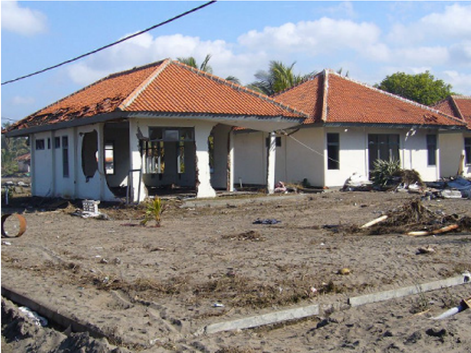
Fig. 4b Damage to buildings near Pangandaran. Note the damaged roof for the building on the left, indicating the height of the tsunami.
