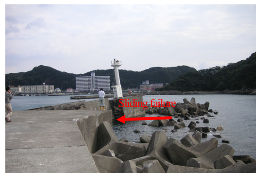
Photo. 2 Sliding failure of caissons at Susami fishery port
