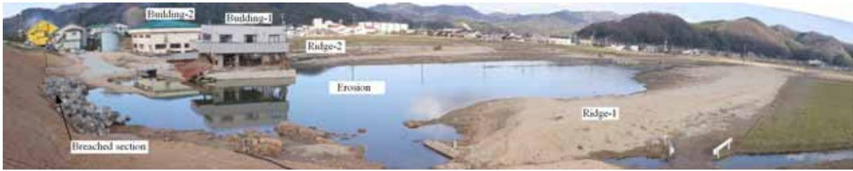
Photo. 1 Panoramic view showing consequences of levee breaching at Tachino, as of December 22, 2004
