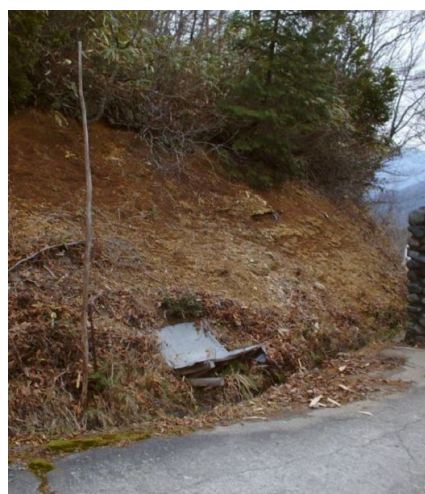
Photo 1 Bare slope at No.1 plot
