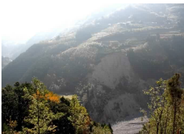
Fig. 14 Topographic features before and after the landslide (above) and an oblique view of Shimato slide.
