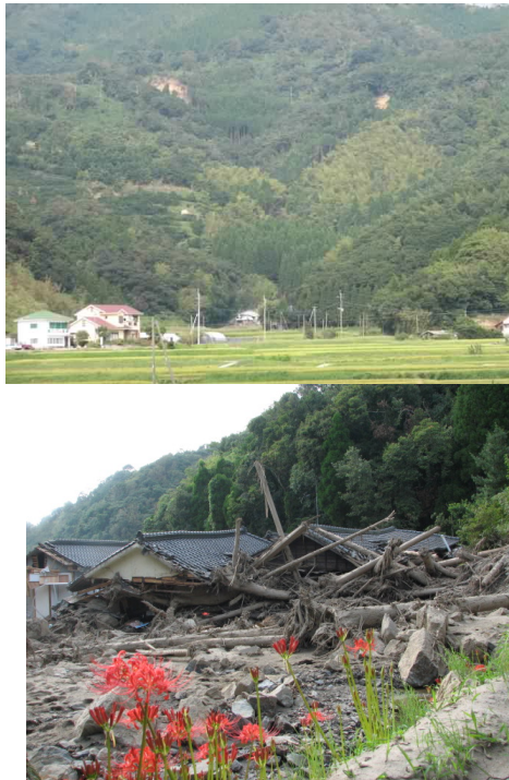
Fig. 3 Slope failures at Shinmido. Landslide scars (above) and the damaged house at the top of an alluvial cone (below).
