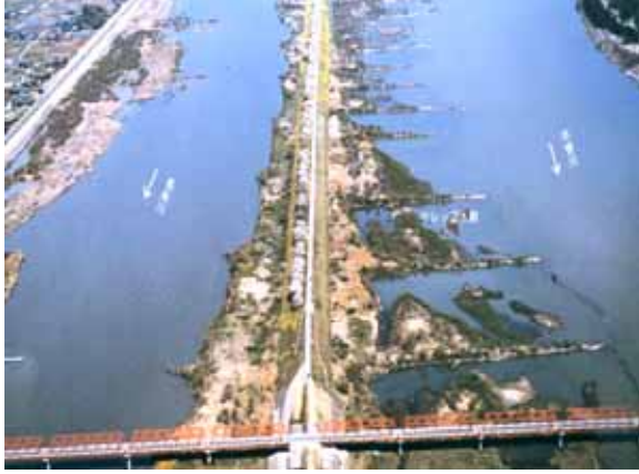
Fig. 7 A series of spur dikes normal to levee between the Kiso and Nagara rivers (adapted from a brochure of the Kiso River Office, MLIT)
