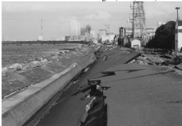
Fig. 1 Typical damage to river embankments (Yodo river embankment during 1995 Hyogoken Nambu earthquake) (after Ozutsumi et al, 2002)
