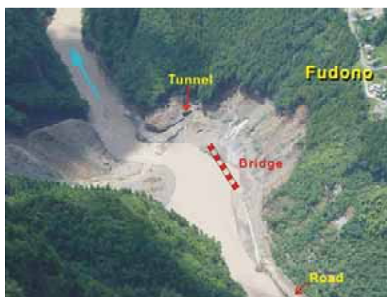
Photo 6 Oblique aerial view of the Fudono area after the landslide (photo by Shikoku Regional Development Bureau, MLIT, Japan)
