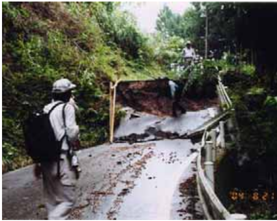
Photo 7 Subsidence on the left hand side of the landslide locating on the upper part of the Azue landslide scarp (yellow dashed region in Photo 5)
