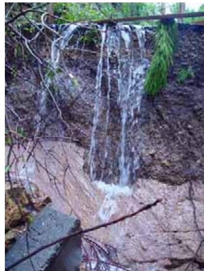
Photo 8 Exposure of the sliding surface beneath the old landslide. The materials above/below the sliding surface are weathered green stone
