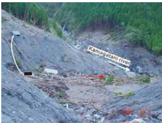
Photo 11 A displaced concrete block from the soil-conservation (check) dam (Black area outlined by the broken white line) on the slope opposite the landslide source (Red arrow: downstream of the valley; White curved arrow: move direction of the block)
