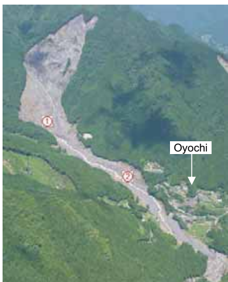
Photo 2 Oblique aerial view of Oyochi landslide (photo by Shikoku Regional Development Bureau, MLIT, Japan)
