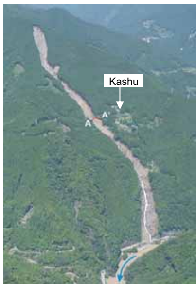
Photo 4 Oblique aerial view of Kashu landslide (photo by Shikoku Regional Development Bureau, MLIT, Japan)
