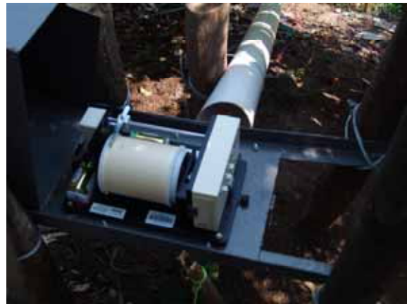
Figure 8 Extensometer installed in Shuping landslide The deformation is recorded on the rolled paper (left) and also saved in a memory (right box)
