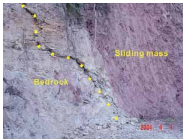
Figure 4 Deformation situation at the right boundary of Block-I outcropped at a roadside
