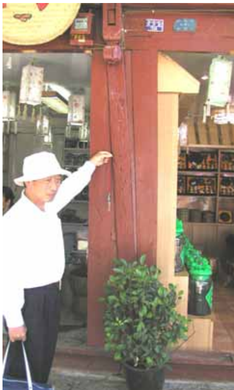
Fig. 2 Shop pillar with a residual tilt of seismic damage, reinforced with wedge boards on the both side, in the Old Town of Lijiang (a World Cultural Heritage), Lijiang, northwestern Yunnan.
