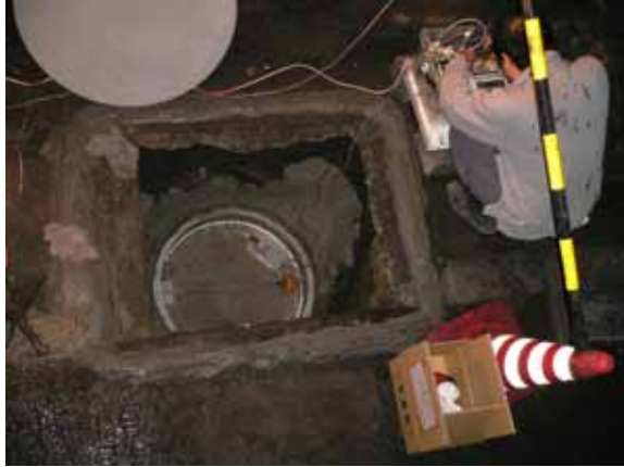
Photo 3 The setting of the cylinder of the short span strainmeter into the hole.
