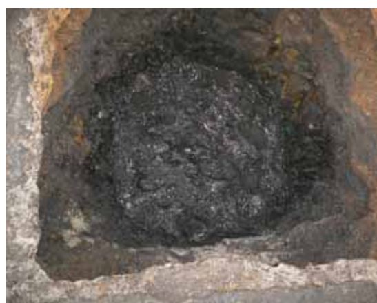
Photo 2 Hard rock in a hole excavated for setting the short span strainmeter.
