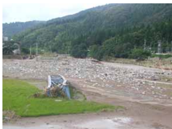
(f) Railway bridge washed away
