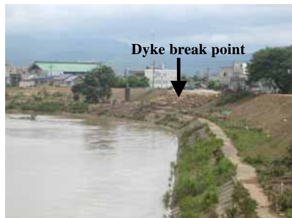
(a) Dyke break point along the Asuwa River.
