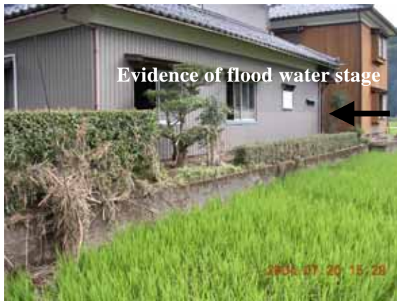
(a) Evidence of flood water stage
