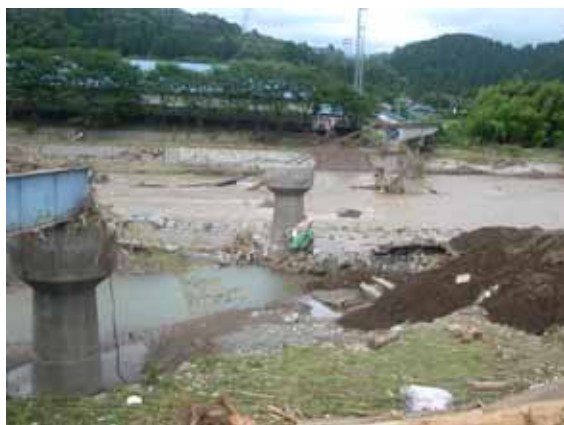
(e) Collapsed railway bridge
