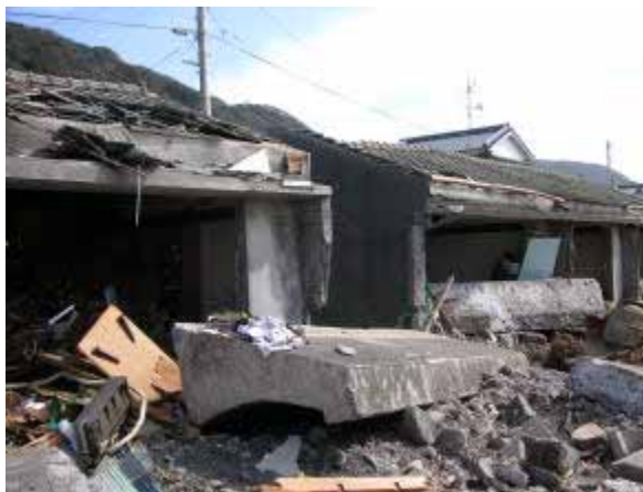
Photo 2 Situation of houses plunged by collapsed parapets
