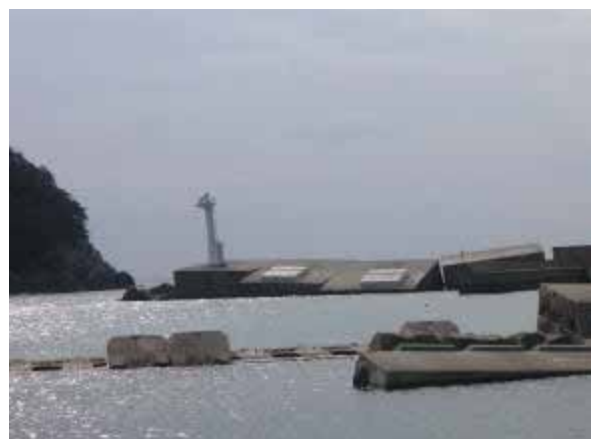
Photo 3 Damaged breakwaters at Susami fishing port
