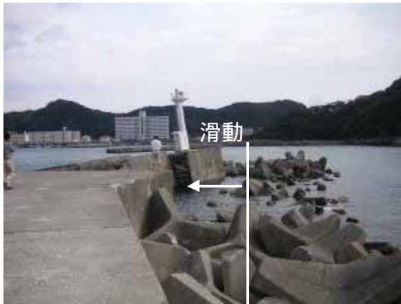
Photo 4 Sliding of caissons
