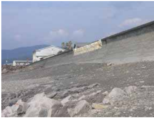
Photo 1 Damaged seawall viewed from sea side
