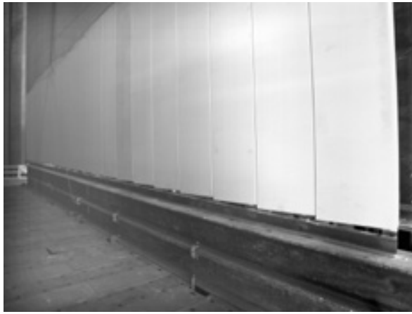
(a) Inclination of ALC Panels (1/25 rad Drift)
