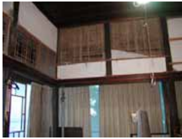
Fig.15 separation of hanging wall (NMH)
