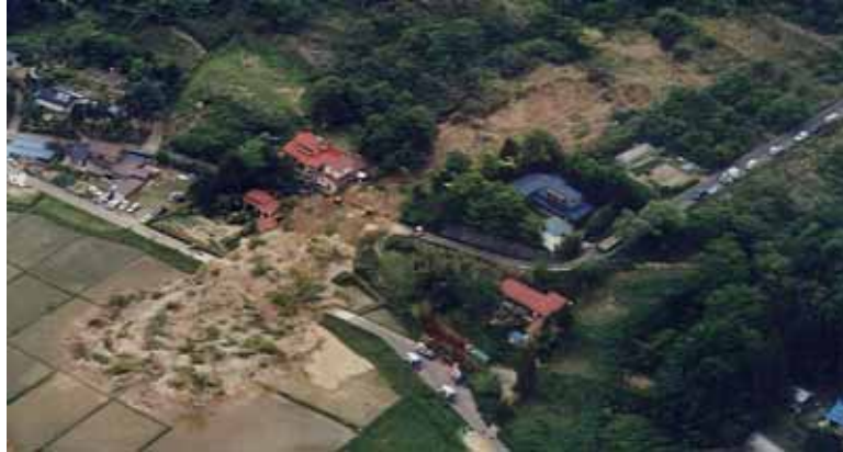
Fig. 9 Oblique side view of the landslide (Photo courtesy of Kokusai Kogyo Co., Ltd).
