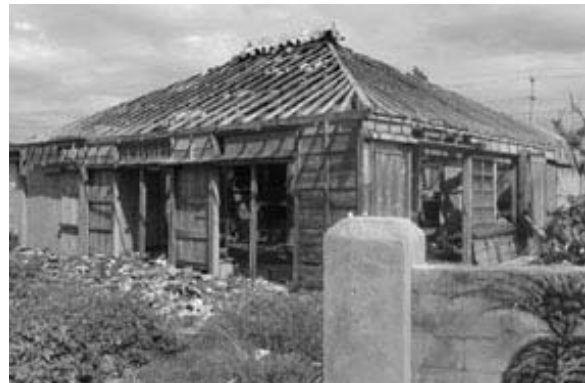
Photo 5. Completely destroyed wooden house.
