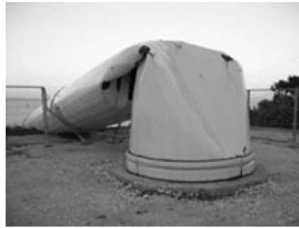
fallen tower of wind turbine
