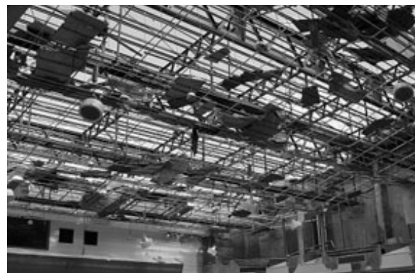
Photo 6. Blow off of a gymnasium roof.
