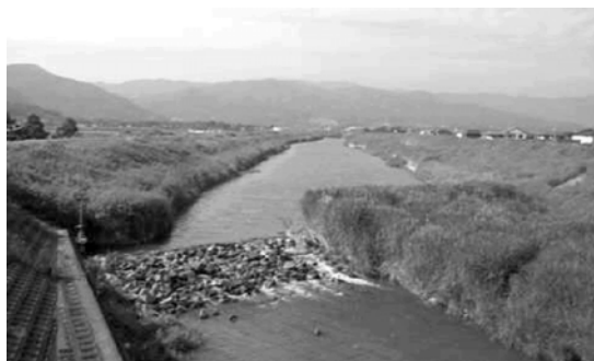
Photo 1 Rubble mound weir in Jobaru River
