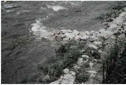
Photo 3 Rubble mound groin in Akechi River
