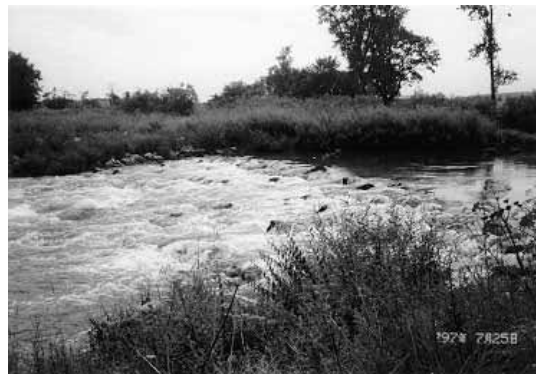
Photo 2 Rough ramp in River Danube
