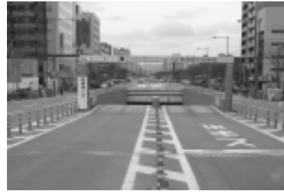
Fig.16 Entrance of underground parking lot
