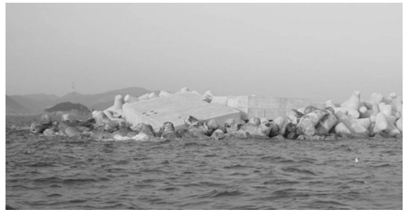
Photo.6 Breakwater damage at the tip
