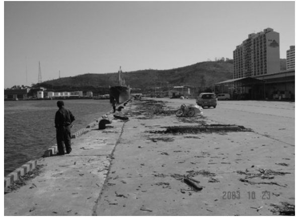
Photo.15 Seohang Quay Wall
