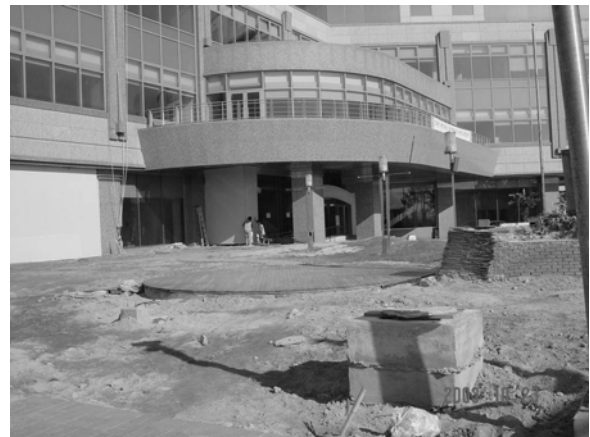
Photo.2 Damaged hotel at Suyeong
