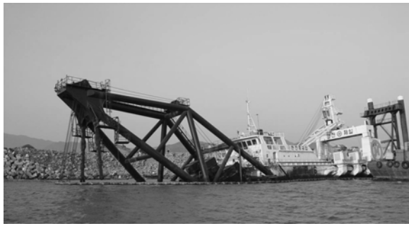
Photo.5 Sunk dredger at Busan New Port
