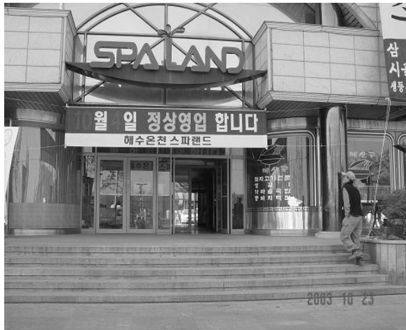
Photo.12 Entrance of Spa Land building
