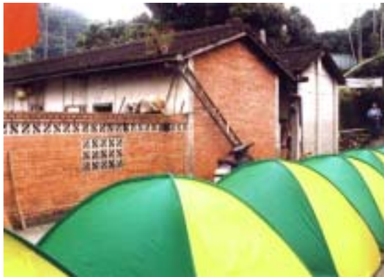
Fig. 1. Undamaged brick wall near northern portion of the Chelungpu fault. Person in far right background is standing on the fault.
