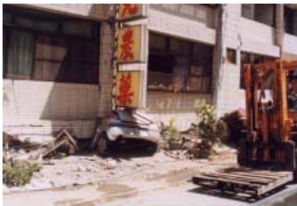
Fig. 2. Collapsed first story of building in ChungLiao Town, near southern portion of the Chelungpu fault, where 95% of the buildings were severely damaged.
