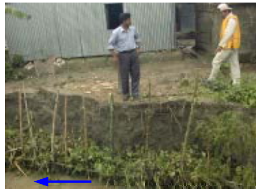
Pile dike along the Jamuna (Klaassen, 2002).
