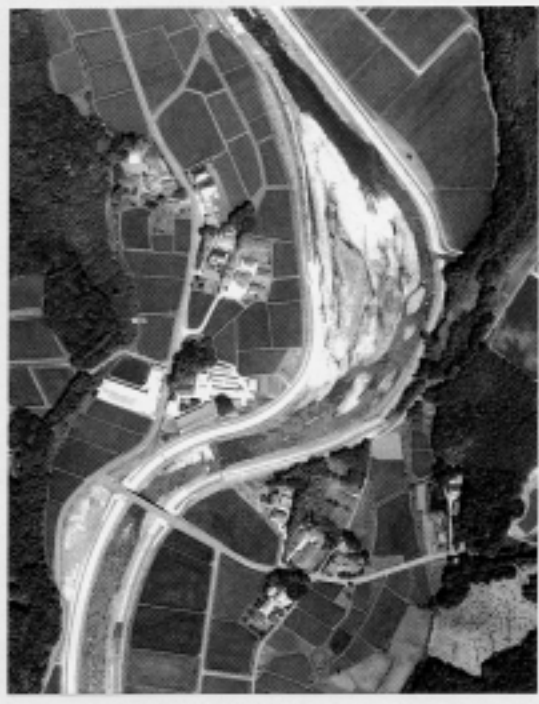
Photo 8 Aerial photographs taken after the river improvement work around the curved channel in upstream area of Kyowa bridge
