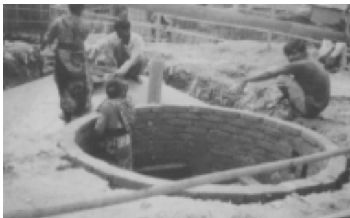
Photo 1 Constructing Bio-gas Plant
