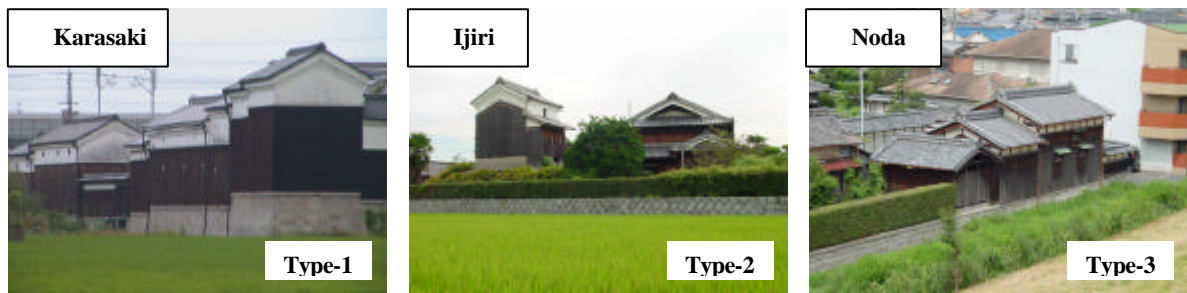
Photo.3 Three types of warehouse with raised base; Type-1 has some stages called as “Rennritsu Dangura”, Type-2 is an isolated warehouse called as “Koritsu Dangura”, and Type-3 is a combined with “Fukugou Dangura”.
