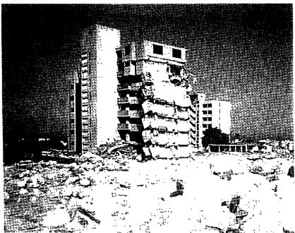
Photo 8 A building destroyed by debris flow
