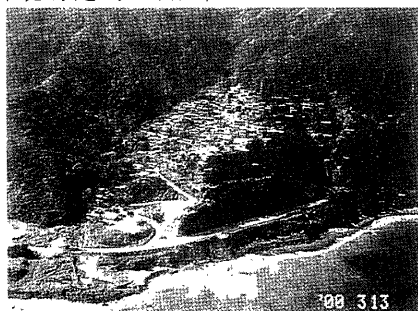
Photo 2 Many houses locate on steep slope
