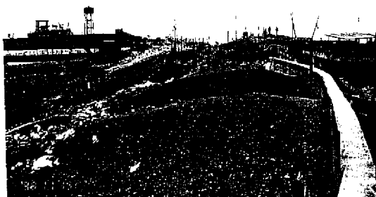
Photo 12 Breach point after the disaster at Jiujiang
