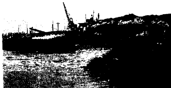
Photo 10 Breach of a dyke at Jiujiang
