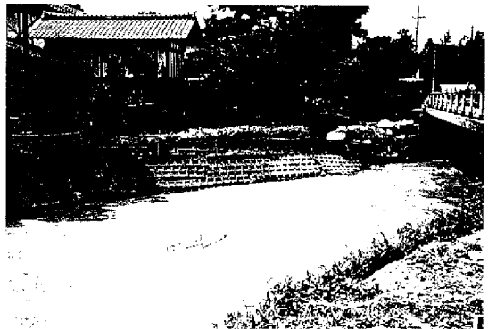
Photo 6 Damaged revetment along the outer embankment
