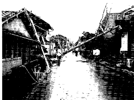
Photo 12 Scene along a street just after typhoon hitting (by Shinjo town)
