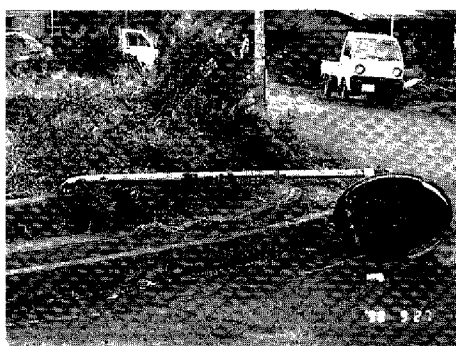
Photo 16 Fully fell down traffic mirror (Shinjo town)
