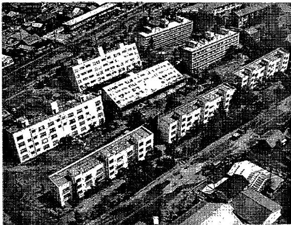
Photo 2 Overtum of Kawagishicho apartment house due to Niigata Earthquake
