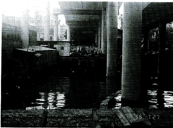
Photo 2 Urban drainage in Guangzhou city
