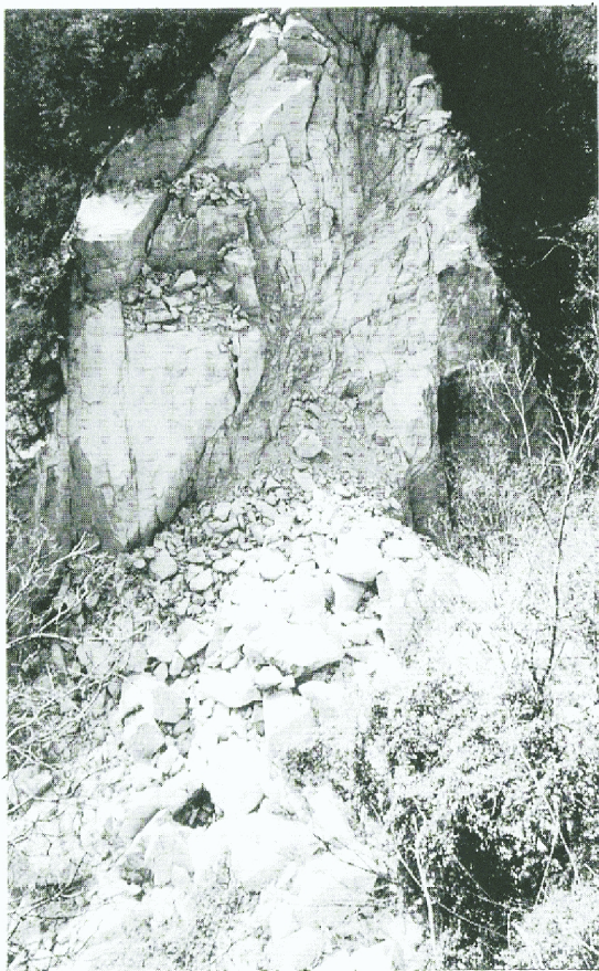
Photo. 1 Failed surface and deposited materials
