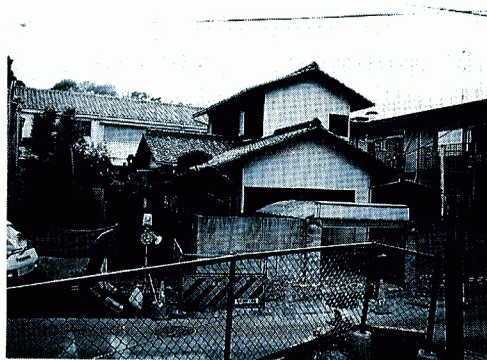
Photo 1 Earthquake damaged House SU (Nishinomiya).
