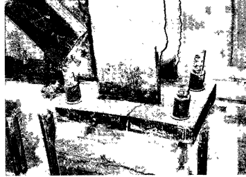
Photo 1 Fracture of base plate observed in the 1994 U.S. Northridge Earthquake
