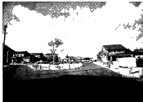
Photo 3. Rebuilt houses at a resettlement site
