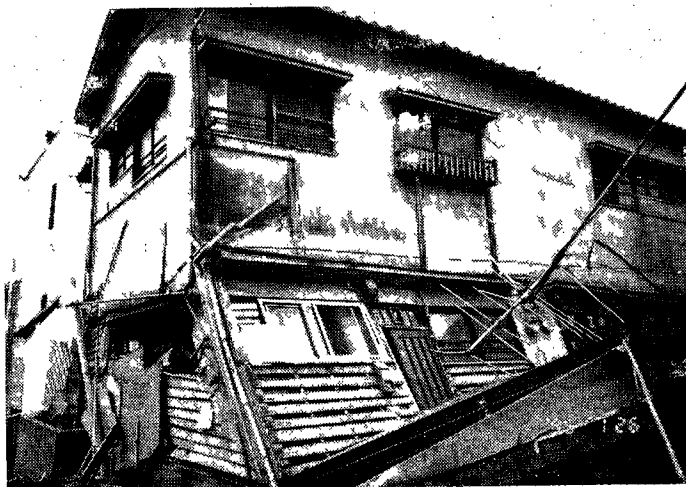
Photo 3 Collapse of inner-connected wood apartmenthouse.
