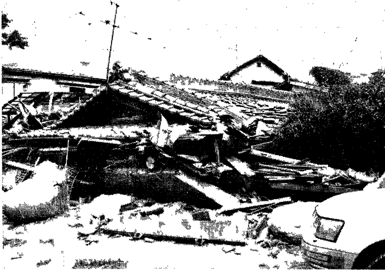
Photo 1 Collapse of a wood house with heavy Japanese roofing tiles on cementing soils.
