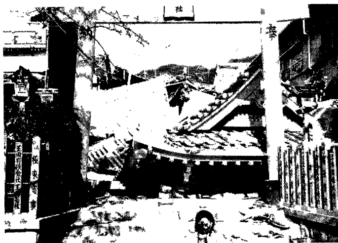
Photo 5 Collapse of a shrine with heavy roofing.
