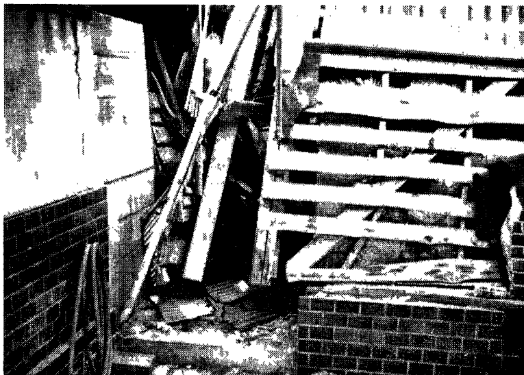
Photo 6 Failure of poor column-to-base connection.
