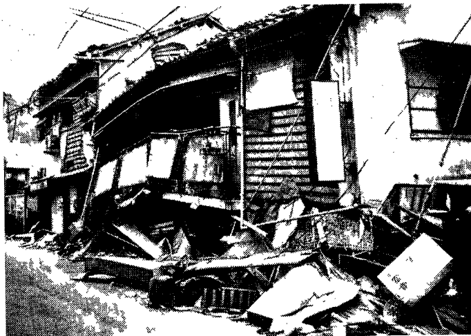
Photo 4 Collapse of wood houses with retail space.
