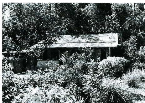
Photo 2 Restoration house at Gobleng village
