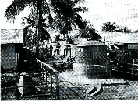
Photo 11 Water tank at Uring Baru
