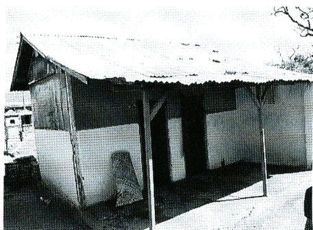
Photo 1 Restoration house at Pengastulan village
