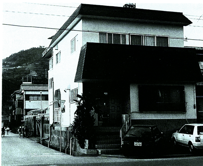
(a) fill-up ground
