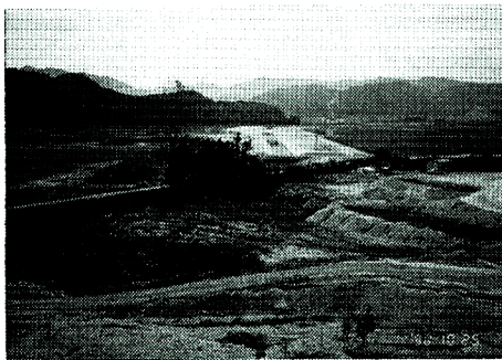
Photo. 6. The Ono River diversion channel under construction.
