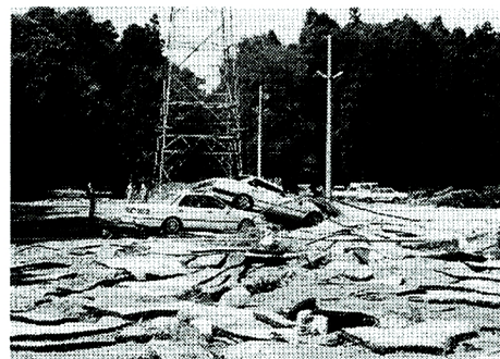
Photo. 9. Situation of the parking area destroyed.
