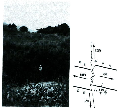
Photo 15 A surface faulting at the Calasigan pass (180 km from Manira).
