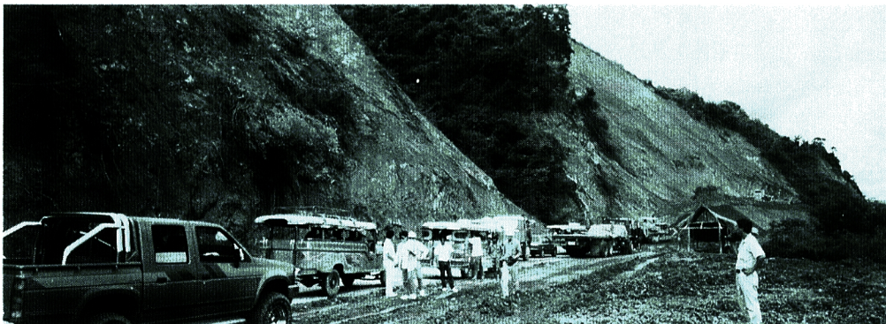
Photo 12 Slope failures along Route 5 (172 km from Manira) near the Digdig fault.
