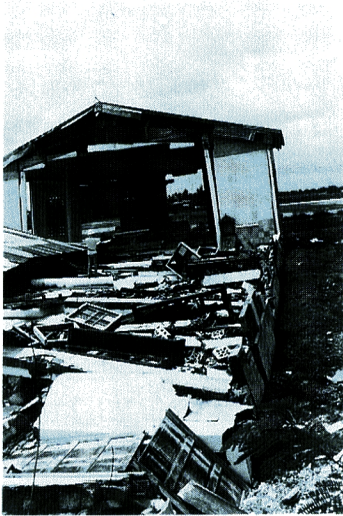
Photo 10 A church collapsed by liquefaction at Pura.
