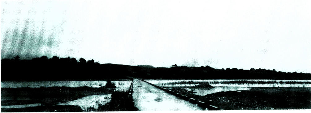
Photo 21 Bato Ferry submerged bridge.
