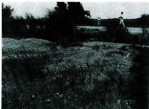
Photo 2 Liquefaction phenomenon in the vicinity of Rizal.
