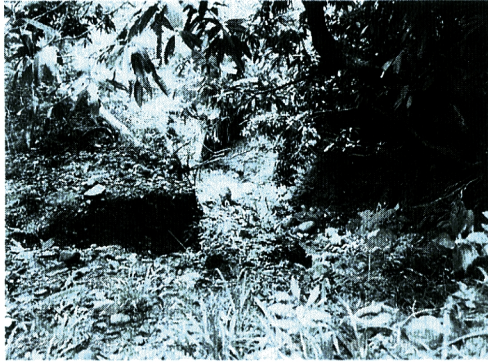
Photo 3 Surface faulting in the vicinity of Rizal.
