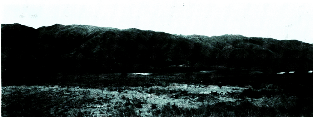
Photo 23 Slope failure toe at Baterya.
