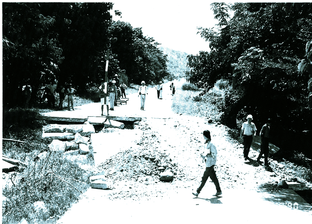
Photo 1. View toward the east showing offset of a branch road in Digdig. Leftlateral offset is 4.8 m and vertical one is 1.5 m.
