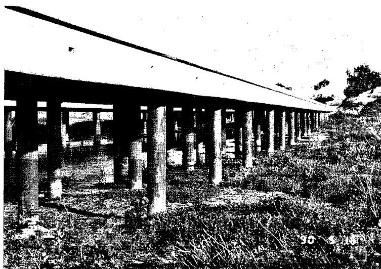
Photo. 26. Reconstructed Struve Slough Bridge (photographed on 5/16/90).
