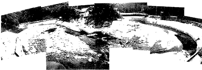
Photo. 9. Collapsed revetment along the outer bank in a curved channel in the Igawa River (W bend, see Fig. 3).
