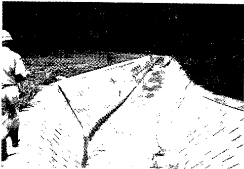
Photo. 6. Slightly damaged revetment in the Aokawa River.
